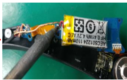
Remove battery wire.
